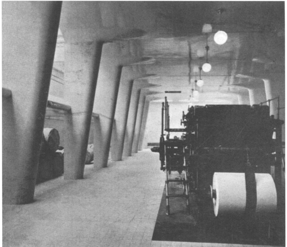
Fig. 1 View of Turun Sanomat Building International Style: Architecture Since 1922 , 1932
